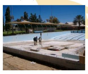
By deepening the pool in a manner that approximately maintained the same volume of water meant that changes to the mechanical plant were not required and the new design resulted in a significant saving for the project.
