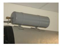
A recent improvement to Solahart's solar hot water technology is an over temperature protection system, otherwise known as OTP. All Solahart systems installed under the Alice Solar City project must have the OTP system fitted. See our FAQ's for more about OTP.
