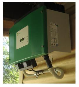
In a typical system, there are two main components – the solar panels (also known as photovoltaic modules or the array) which capture the sun's energy, and a device called an inverter which converts the captured energy into grid friendly electricity. The array is installed on your roof, however ground mounted systems may be possible if installation on the roof is not feasible.
