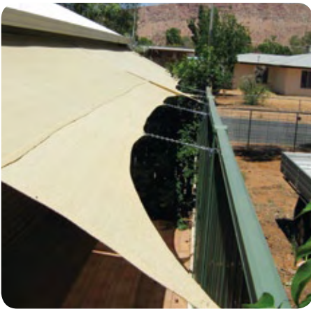
Horizontal awnings used to shade paved or concreted areas
