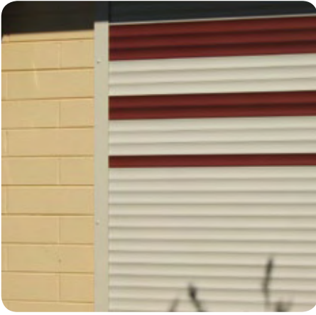
External blinds can be lowered or raised to manipulate the amount of sun
