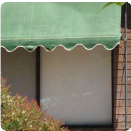
Vertical shading can be lowered to combat higher angle summer sun, but allows lower angle winter sun to warm the house
