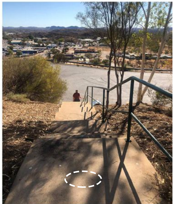
4 - Looking north from the top of the walking steps
