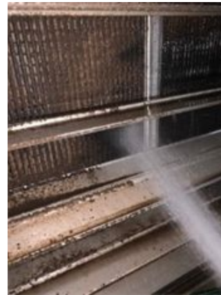
Hosing of internal AHU filters
