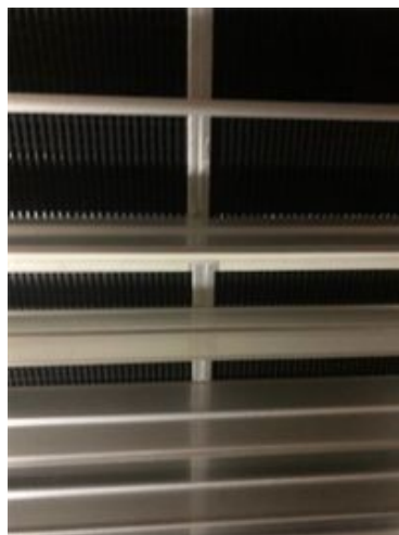
Internal AHU filters after cleaning
