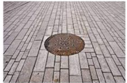
Example of plate levelled into pavers.
